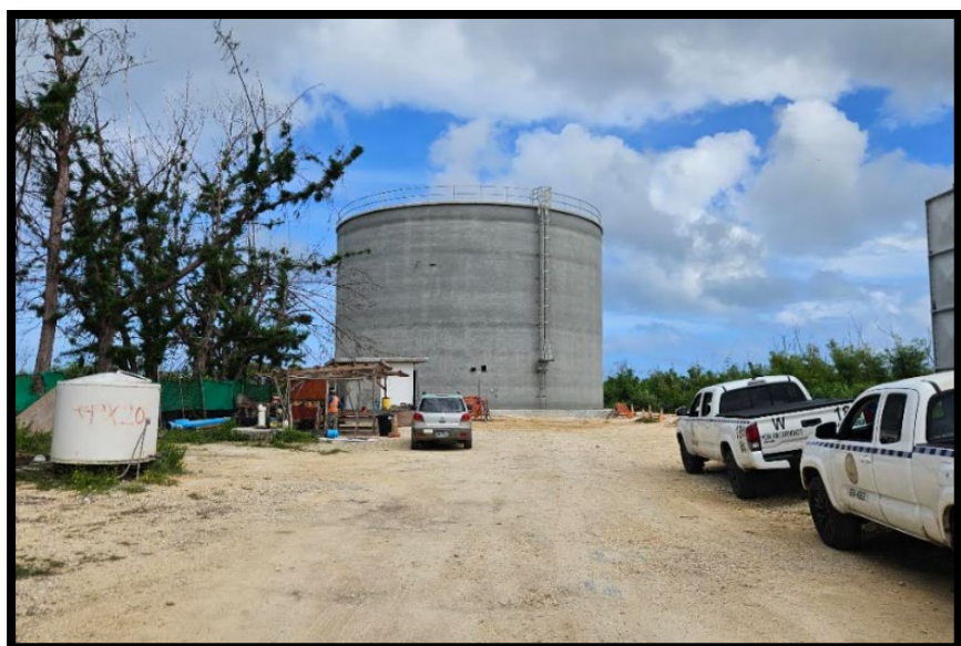
Dandan Water Tank Project Site
