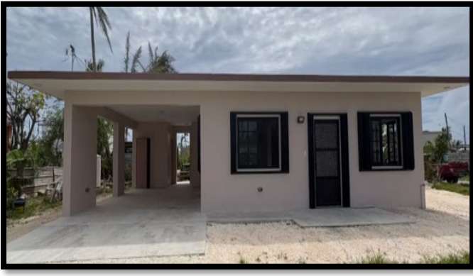
2 Bedroom ADA Re-Construction
