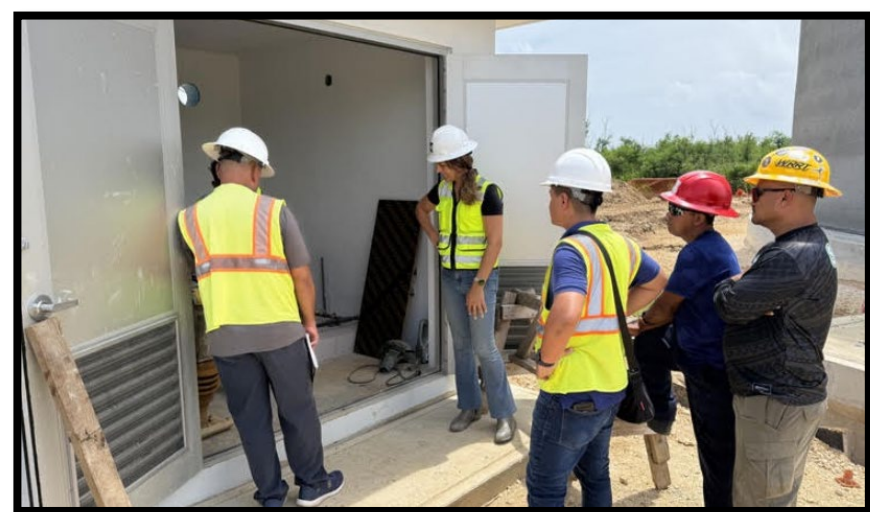
Dandan Temporary Water Tank
