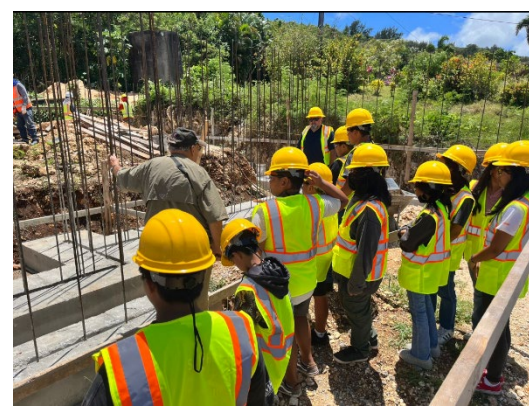
Construction- Onsite Training
