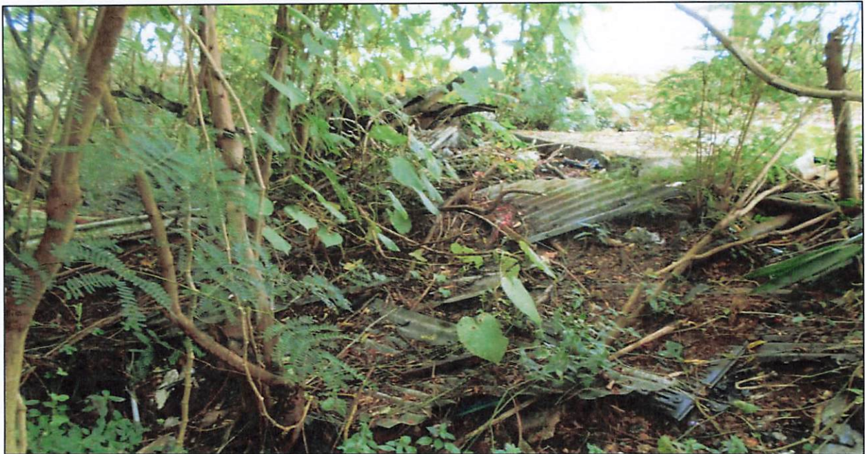
Figure 11: Lot 142-3-3 View north of roofing tins and 2.5 x 2.5 m concrete base (photo: J. Farrugia 2/15/2023).
