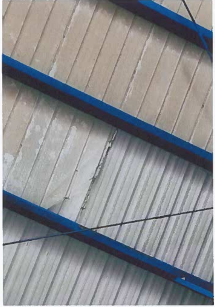
Repaired Section of Roof
