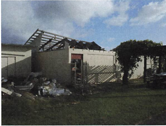
Southeast side of Building E
