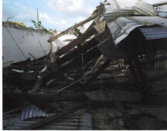
Building E interior
