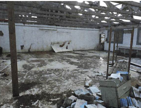
Building D Interior
