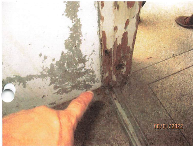
2 ND FLOOR FIRE EXIT DOOR; DOOR JAMB SEVERE TERMITE INFESTED
