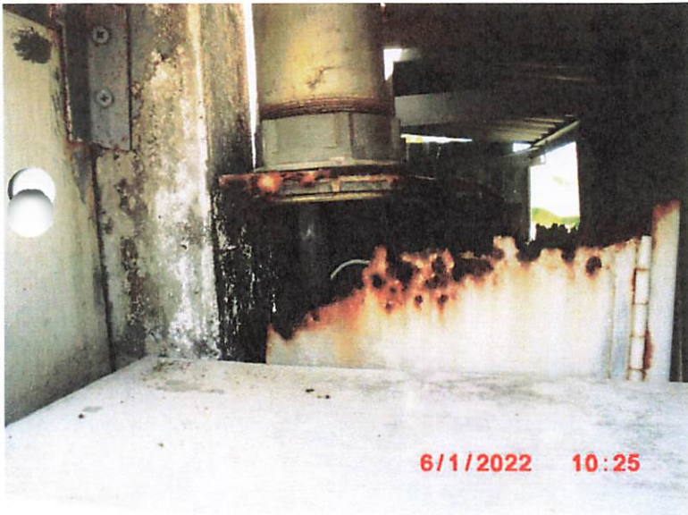
SERVICE UTILITY BOX CORRODED, HIGH RISK, WIRE EXPOSED
