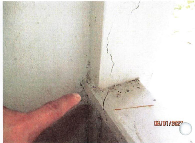
3 RD FLOOR WOOD WALL HAS CRACK
