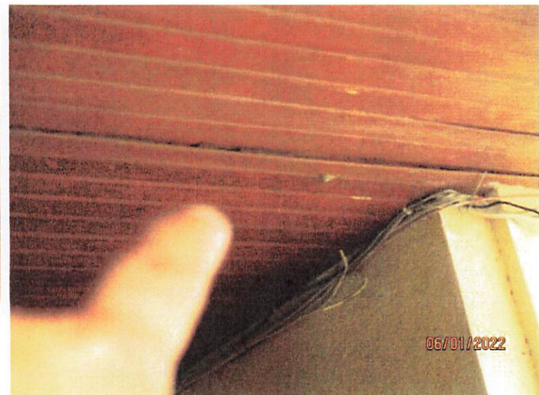
2 ND FLOOR EXTERIOR HALLWAY; CEILING TERMITE INFESTED
