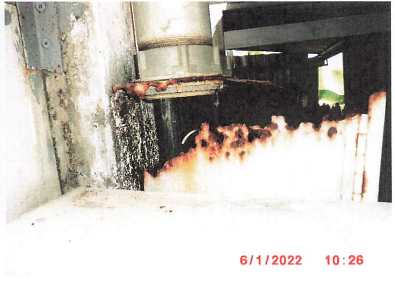
SERVICE UTILITY BOX CORRODED, HIGH RISK, WIRE EXPOSED
