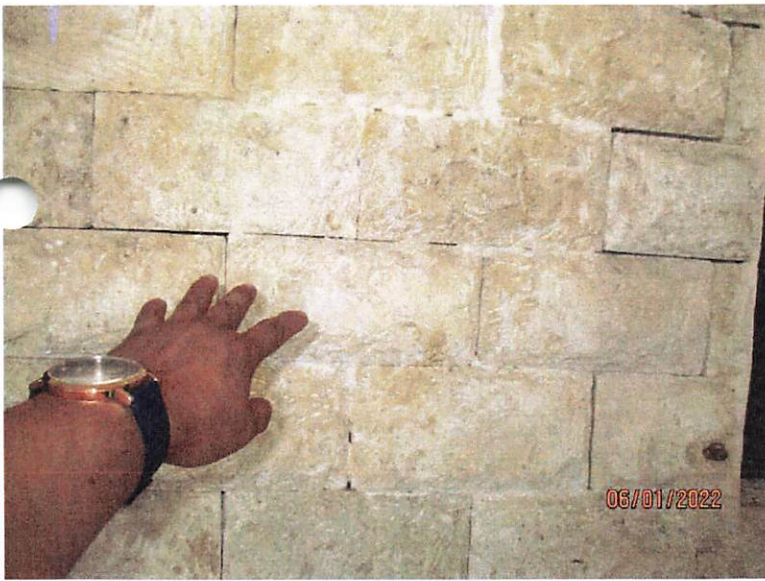
2 ND FLOOR VACANT UNIT NO. 202; WALL MARBLE BRICKS LESS THAN 5% ARE HOLLOW; KITCHEN HOOD RANGE EXHAUST NO COVER
