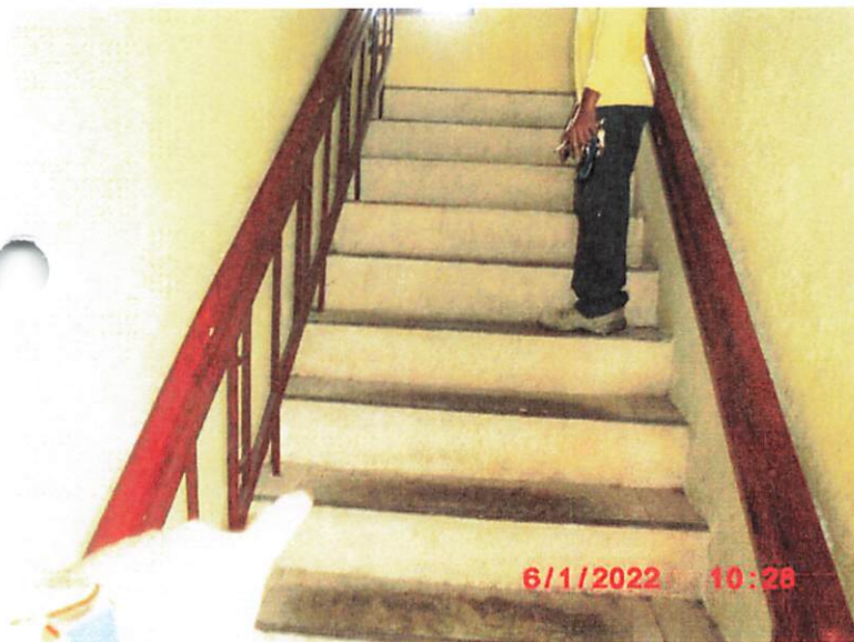
STAIRCASE GOING TO 2 ND FLOOR
