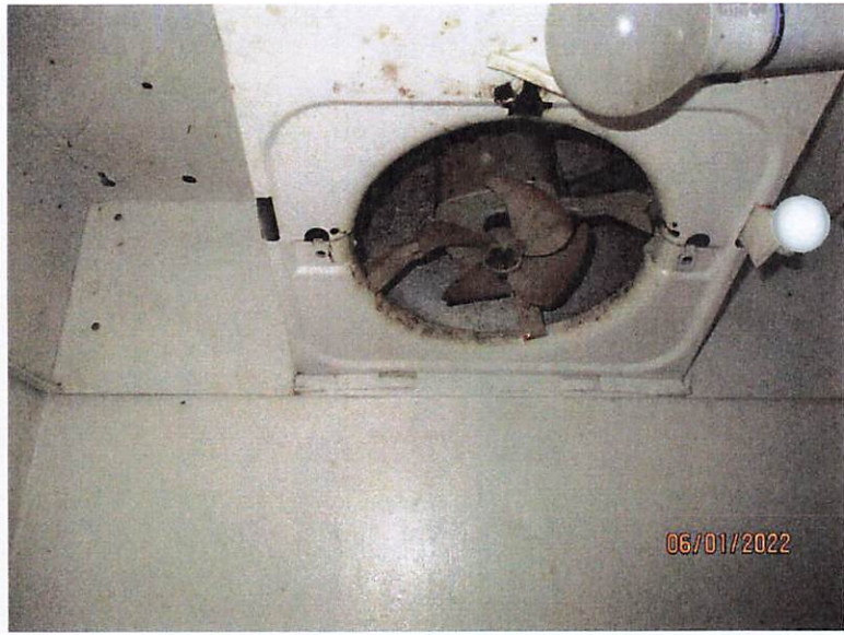
2 ND FLOOR VACANT UNIT NO. 202; WALL MARBLE BRICKS LESS THAN 5% ARE HOLLOW; KITCHEN HOOD RANGE EXHAUST NO COVER
