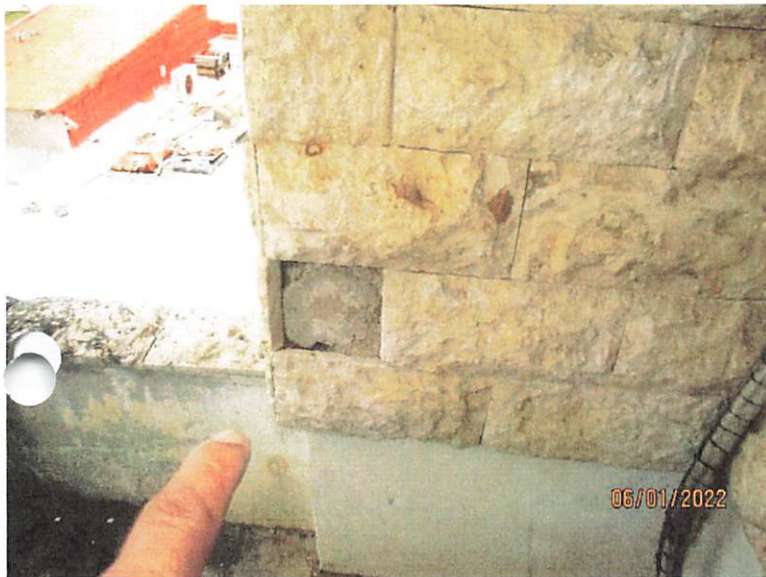
3 RD FLOOR VACANT UNIT; BALCONY WALL MARBLE BRICK 2% MISSING
