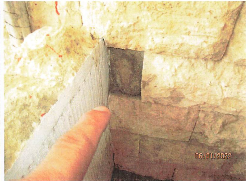
3 RD FLOOR VACANT UNIT; BALCONY WALL MARBLE BRICK 2% MISSING
