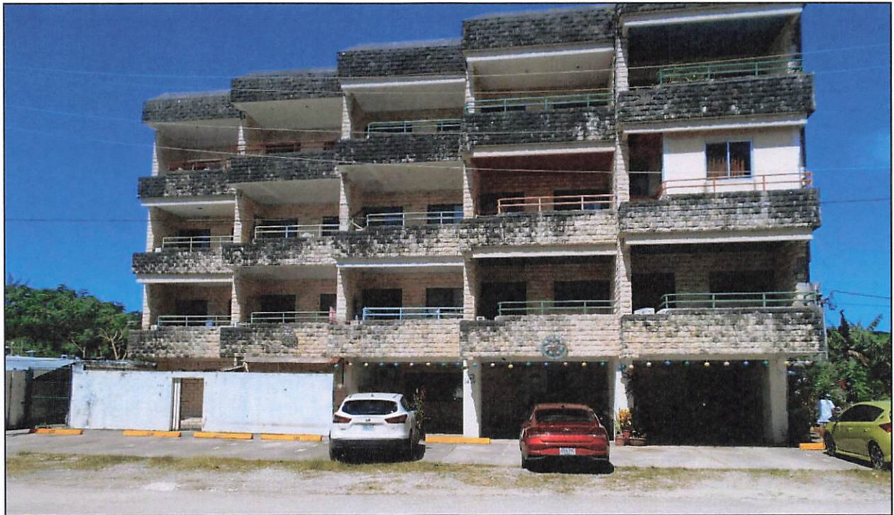
Figure 2: Lot 010 D 12 View north of APE and south elevation of existing apartment building covering nearly the entire lot (photo: J. Farrugia 1/31/2023).
