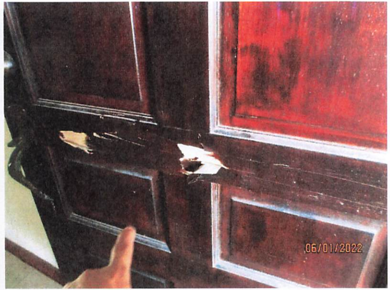
2 ND FLOOR VACANT UNIT NO. 202; MAIN ENTRY DOOR HAS PUNCTURED
