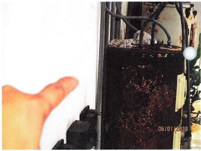
3 RD FLOOR HALLWAY RAILINGS ARE RUSTY; WATER HEATER MACHINE NOT WORKING AND RUSTY CASE
