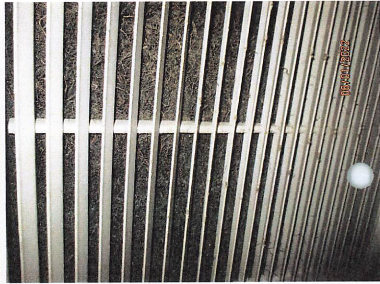
3 RD FLOOR UNIT #3 W/ 2 BEDROOM; CENTRALIZED AIRCON EXHAUST LOTS OF MOLDS
