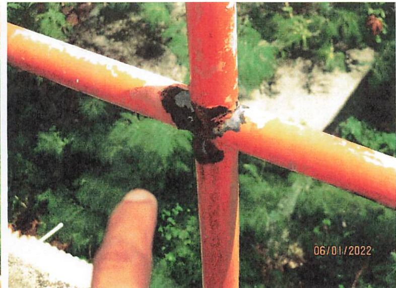
3 RD FLOOR HALLWAY RAILINGS ARE RUSTY AND SOME PORTION MISSING
