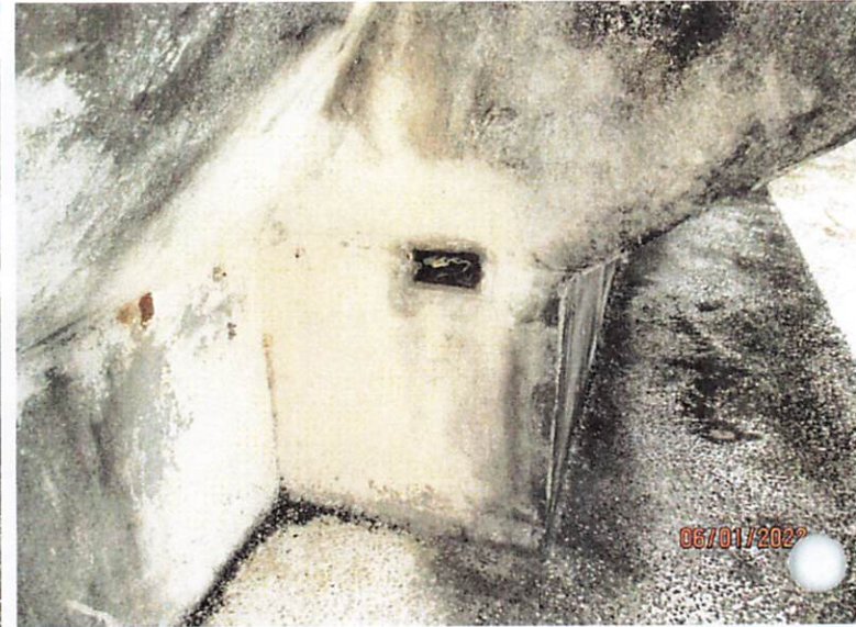
ROOF TOP; LOTS OF DRY ALGAE, LOTS OF UNWANTED STUFF; ELECTRICAL OUTLET ARE OPEN/EXPOSED WIRES
