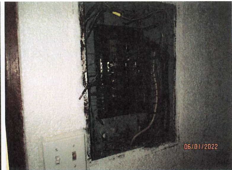
2 ND FLOOR VACANT UNIT NO. 202; BATHROOM LIGHT FIXTURE; ELECTRICAL BREAKER BOX MISSING COVER EXPOSED WIRES
