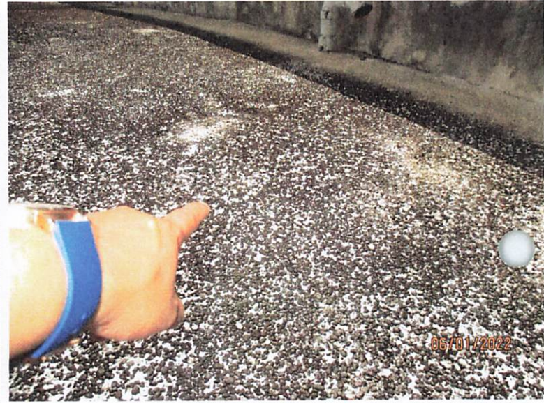
ROOF TOP; LOTS OF DRY ALGAE, SOME PORTIONS ARE HOLLOW.
