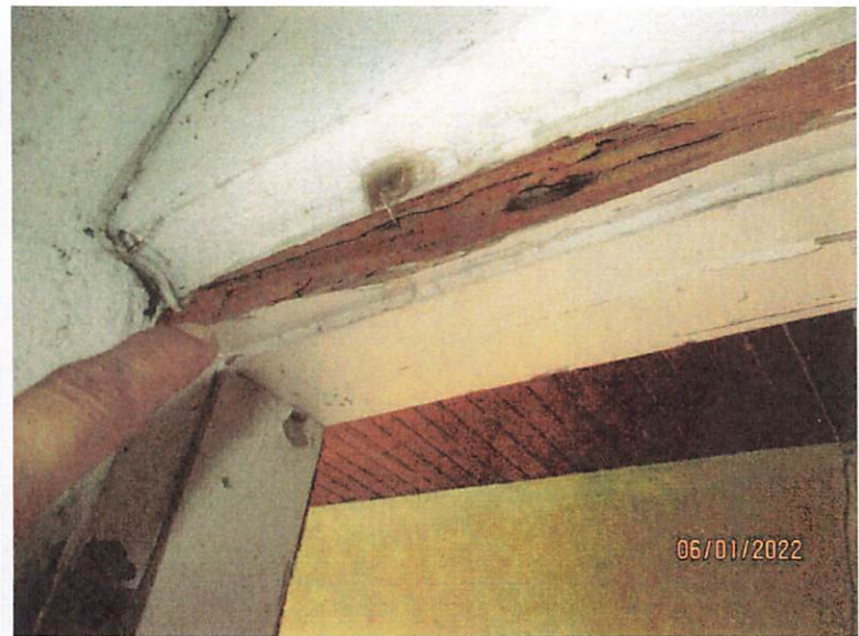
2 ND FLOOR FIRE EXIT DOOR; DOOR JAMB SEVERE TERMITE INFESTED
