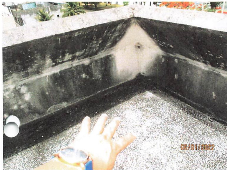
ROOF TOP LOTS OF DIRT STAIN, DRY ALGAE, MINOR CRACK
