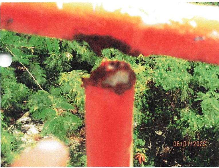
3 RD FLOOR HALLWAY RAILINGS ARE RUSTY; WATER HEATER MACHINE NOT WORKING AND RUSTY CASE
