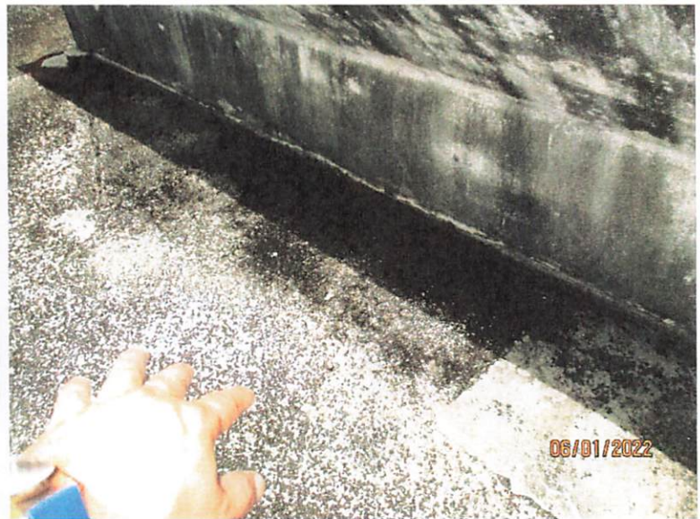
ROOF TOP LOTS OF DIRT STAIN, DRY ALGAE, MINOR CRACK
