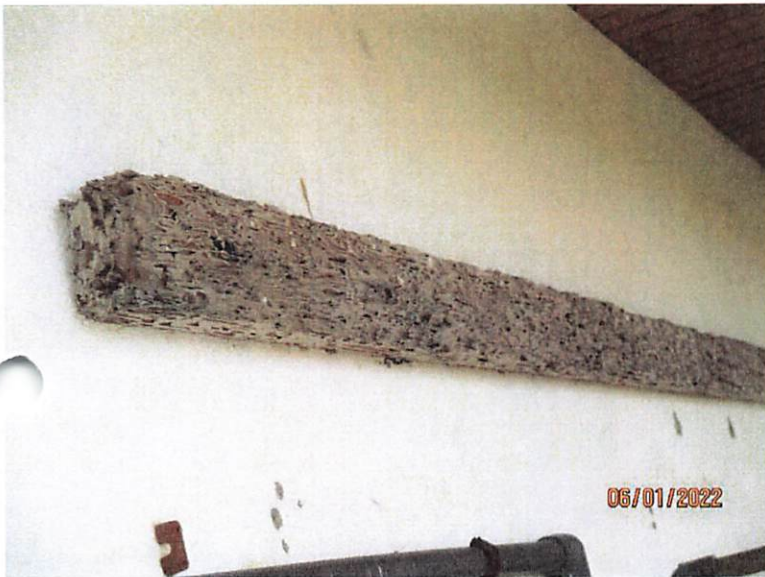
3 RD FLOOR WOOD TRIMMINGS HAS TERMITE INFESTED; WALL HAS CRACK
