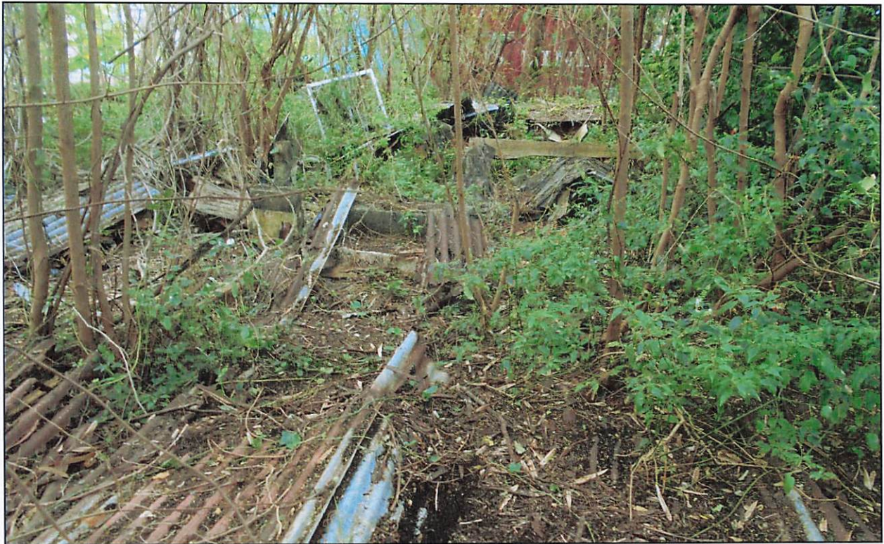
Figure 4: Lot 010 K 417 View south of structural remains (photo: J. Farrugia 2/10/2023).
