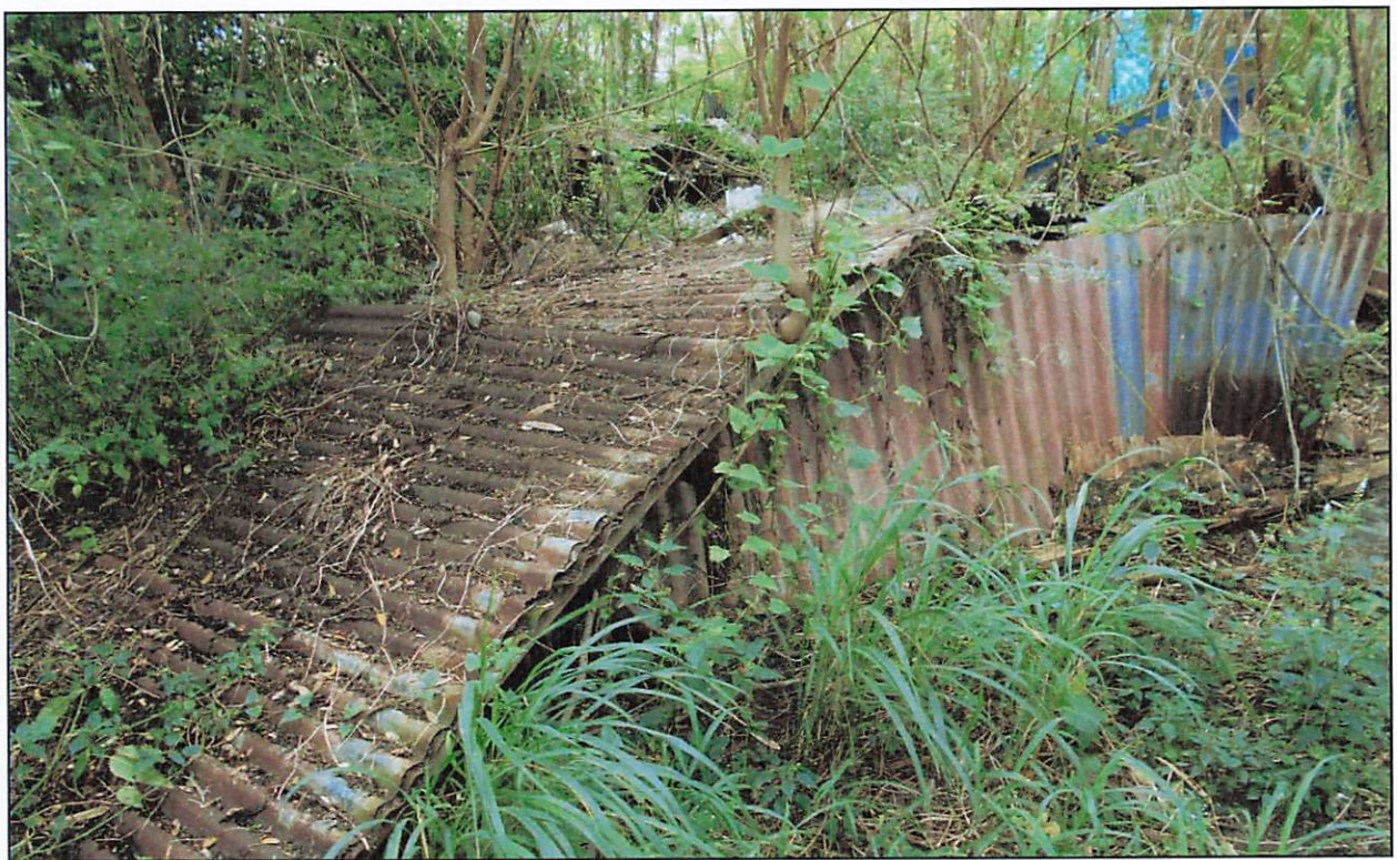
Figure 5: Lot 010 K 417 View southeast of structural remains (photo: J. Farrugia 2/10/2023).
