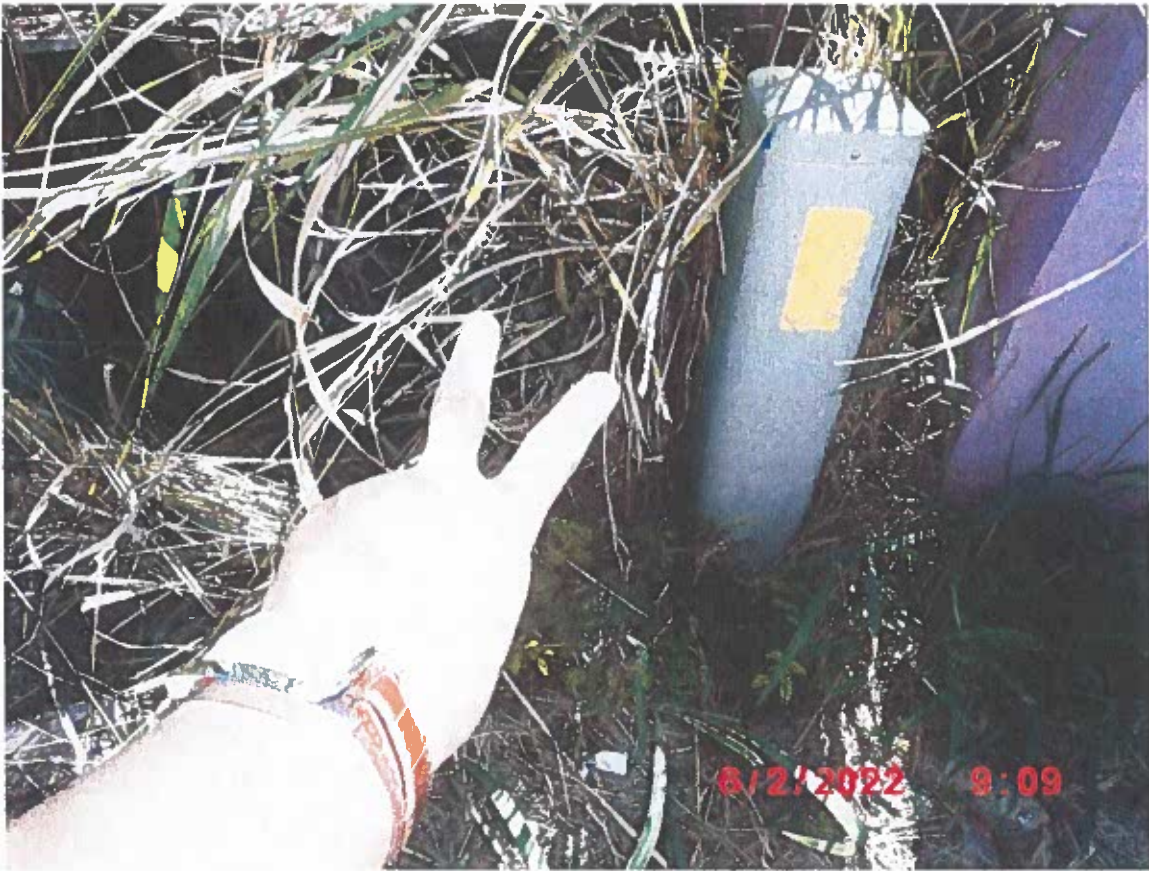
AVAILABLE TELEPHONE POLE
