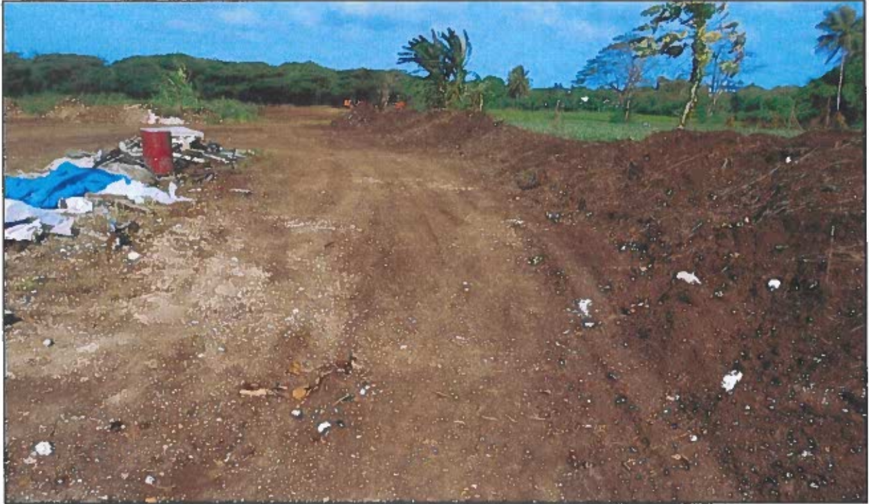
Figure 6: View northeast of push piles along eastern boundary (photo: J. Farrugia 1/24/2023).
