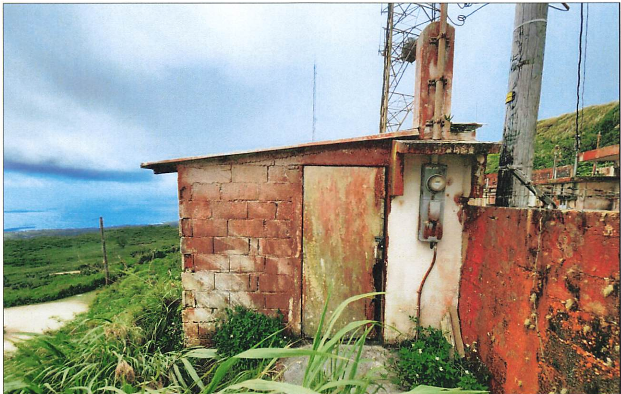
Figure 14: View southeast of northwest elevation of Building 6 (photo: D. Perzinski, 6/15/23).
