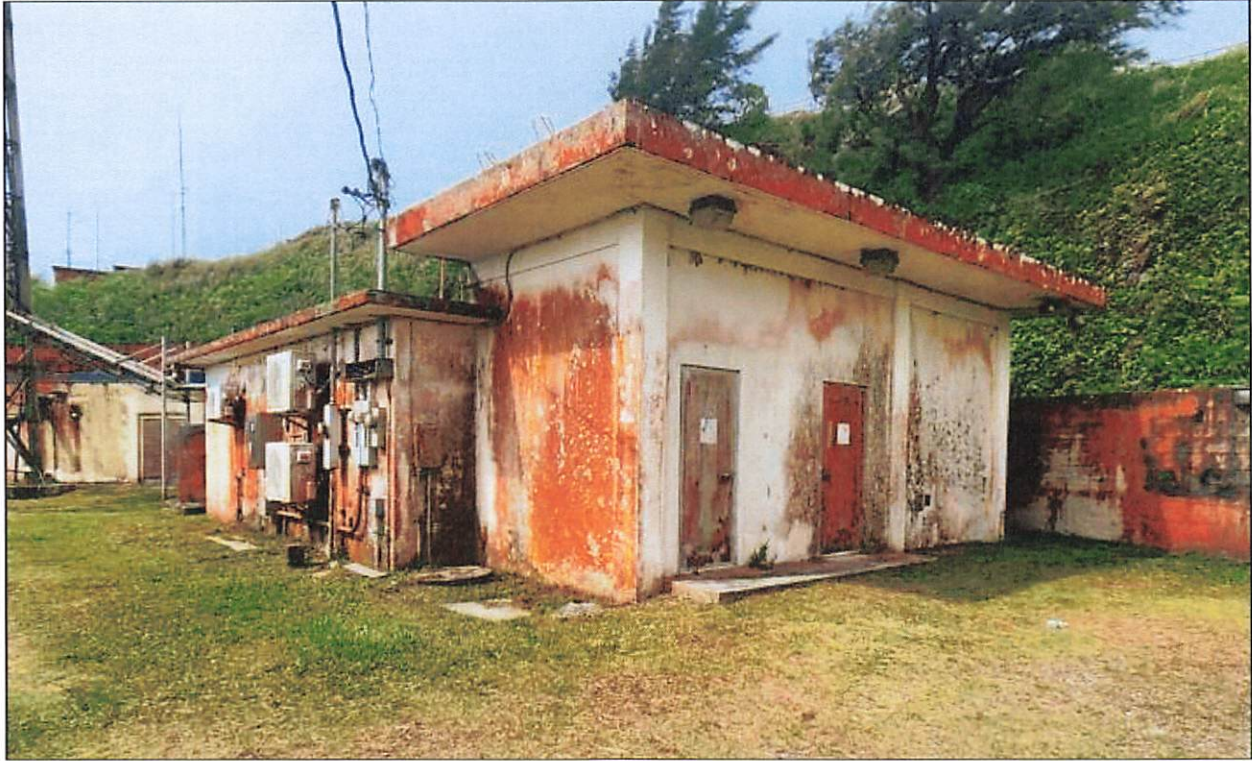
Figure 9: View south of north corner of Building 1 (photo: D. Perzinski, 6/15/23).
