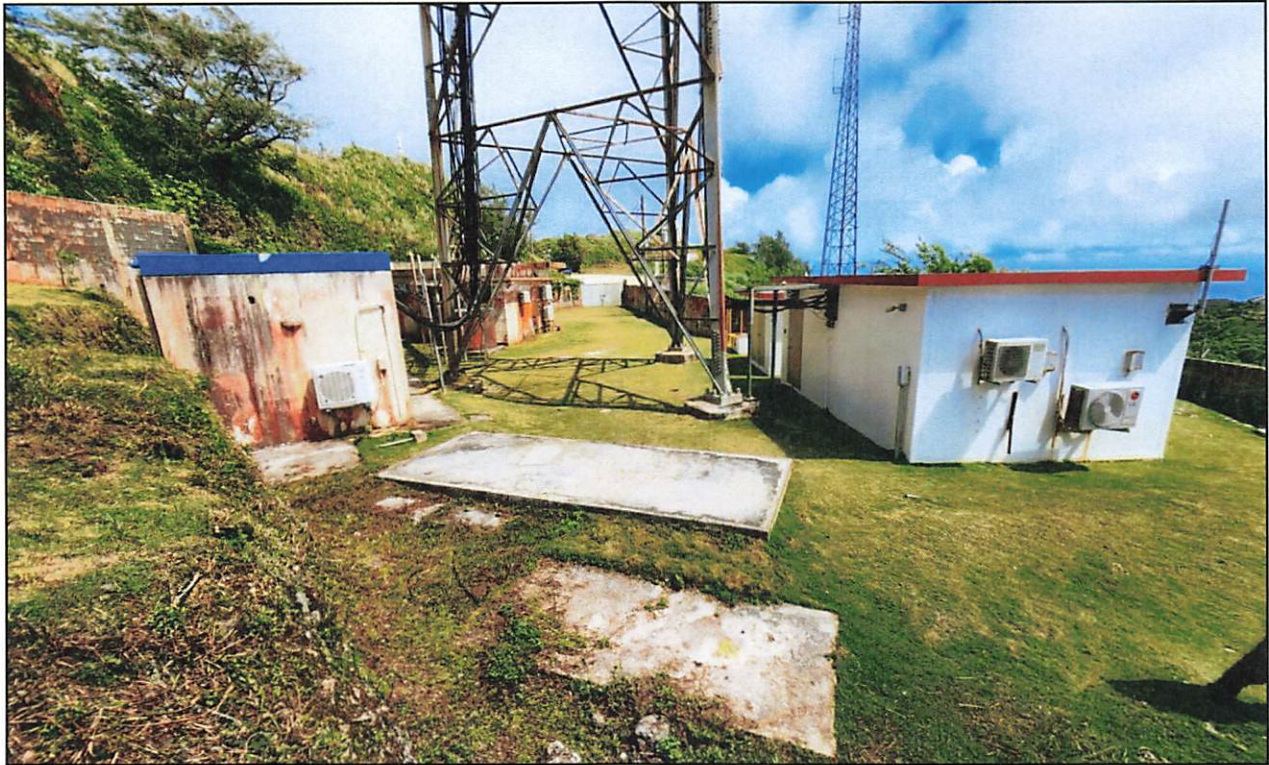
Figure 6: View northeast of tower base and communications buildings from southeast end of compound (photo: D. Perzinski, 6/15/23).
